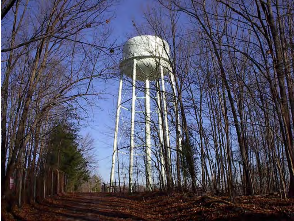
Fig. 4.2. City of Oak Ridge water tank at Parcel ED-6 looking northeast.
