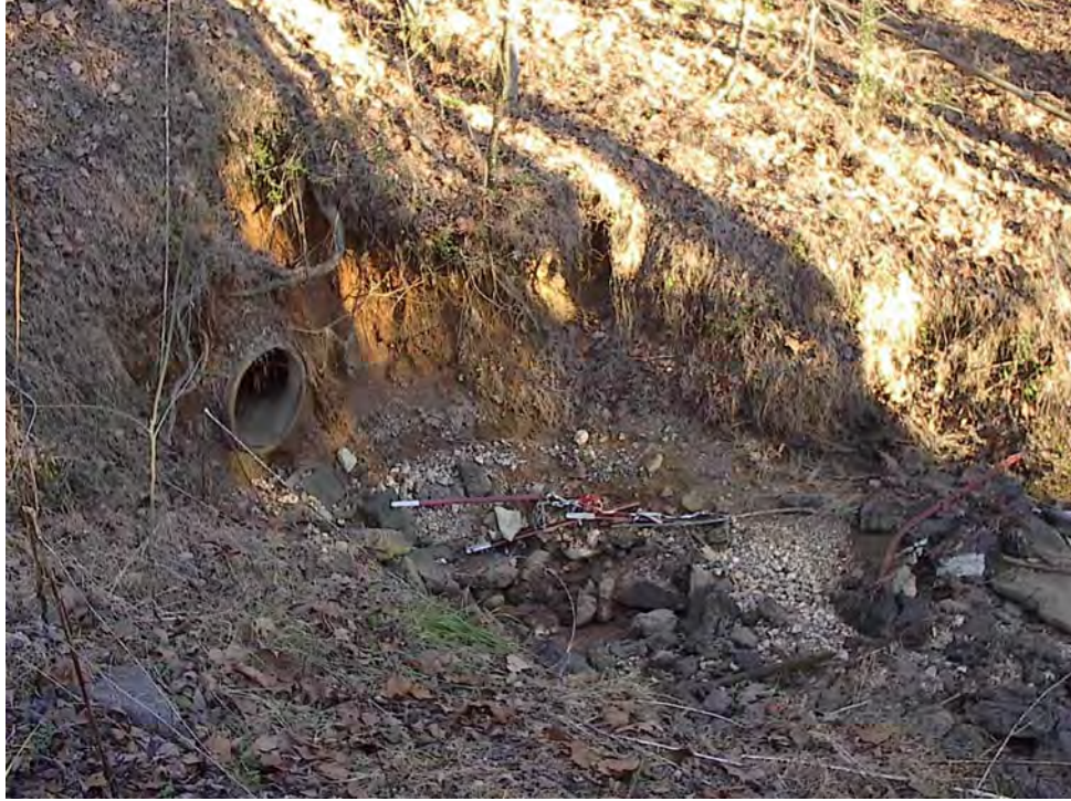
Fig. 5.2. Culvert under East Quarry Road during the dry period.
