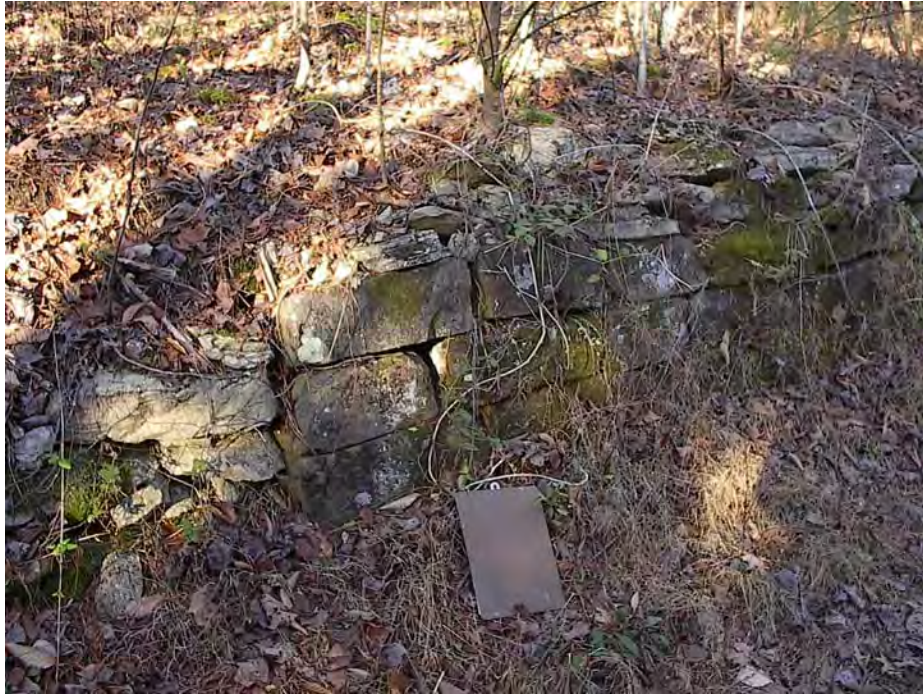
Fig. 5.4. Remnants of a stone wall along East Quarry Road.
