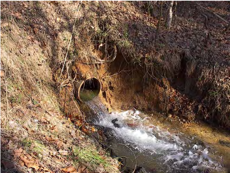
Fig. 5.3. Culvert under East Quarry Road 24 hrs after a precipitation event.
