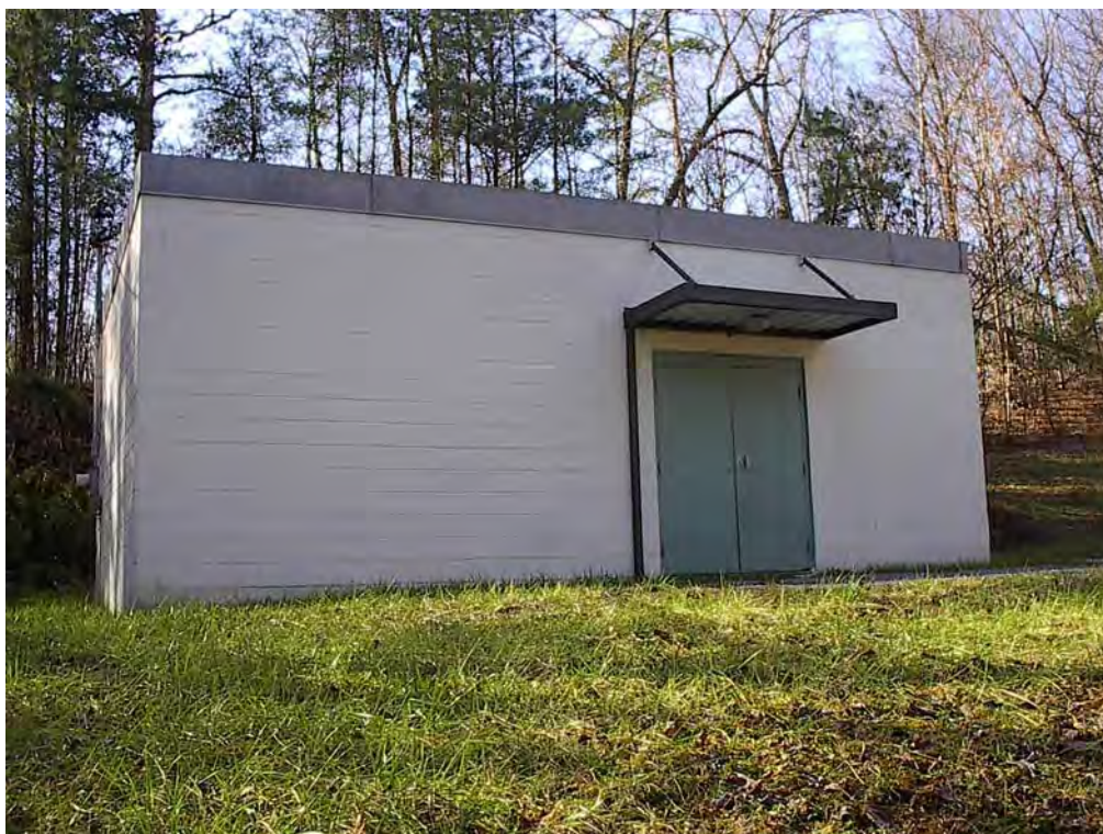
Fig. 4.1. City of Oak Ridge pumphouse at Parcel ED-6.
