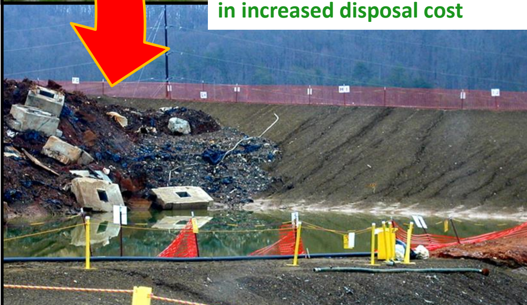
Demolition and remediation waste landfilled in 2002 at the Environmental Management Waste Management Facility (EMWMF)
