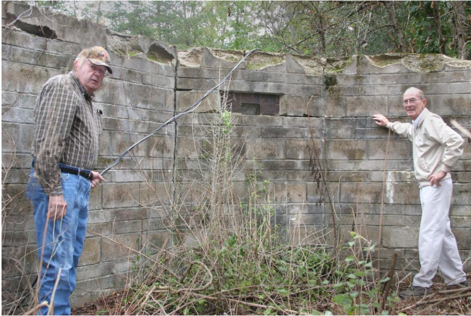
Large concrete block shield built on top of a small hill overlooking the irradiation facility that had lights installed to indicate when the radiation sources were exposed below in the fenced in area
