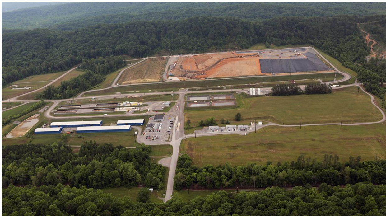
Figure 2. Environmental Management Waste Management Facility.
