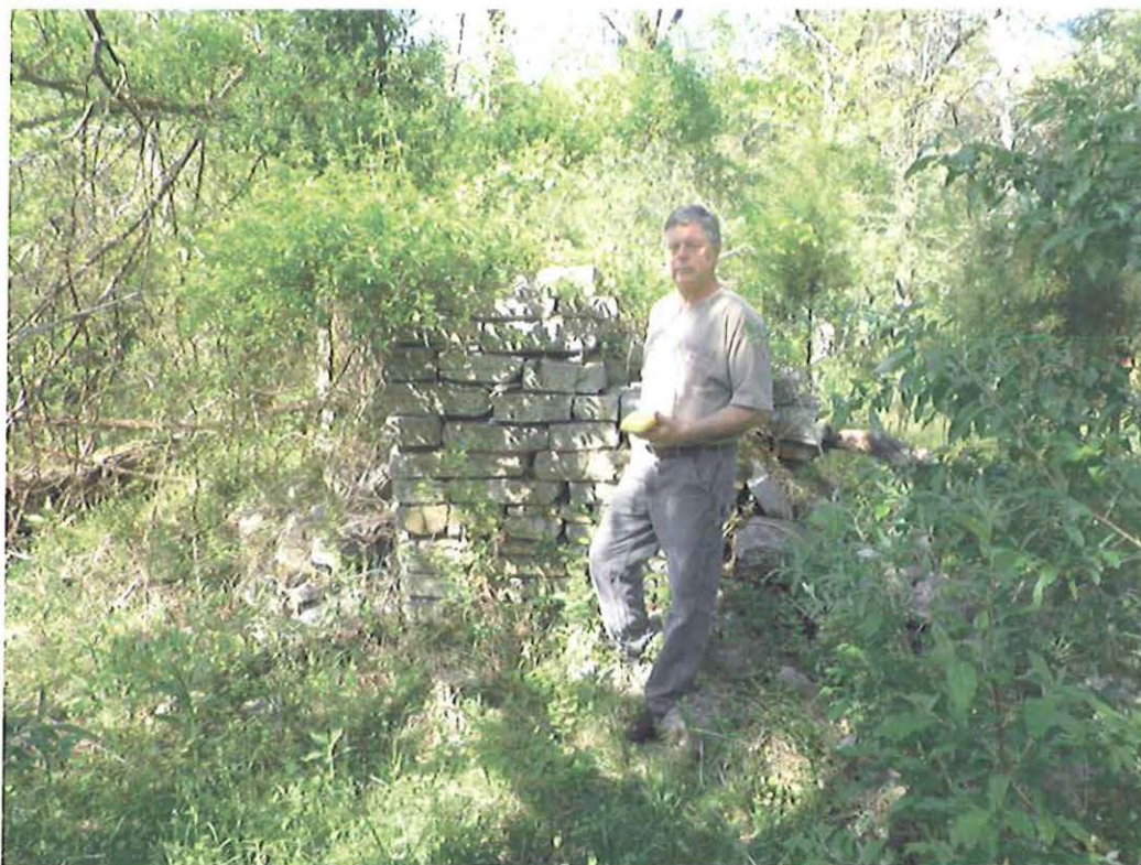
Photograph 21. Stacked stone chimney remnant (Structure 954A) in eastern part of DA 7.
